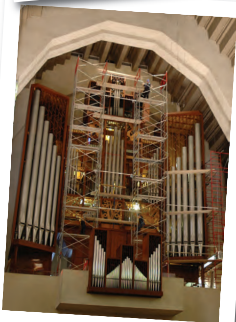
Its sheer size makes it special. It's rare to see 32-ft. pipes on the façade of an organ.
